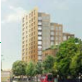
58-70 York Road Under Construction 17 Storeys
