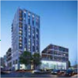
98 York Road Completed 17 Storeys
