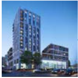
98 York Road Completed 17 Storeys
