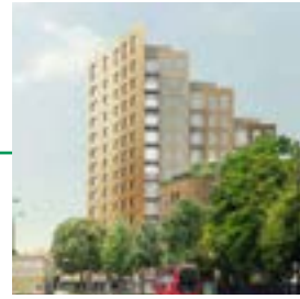
58-70 York Road Under Construction 17 Storeys
