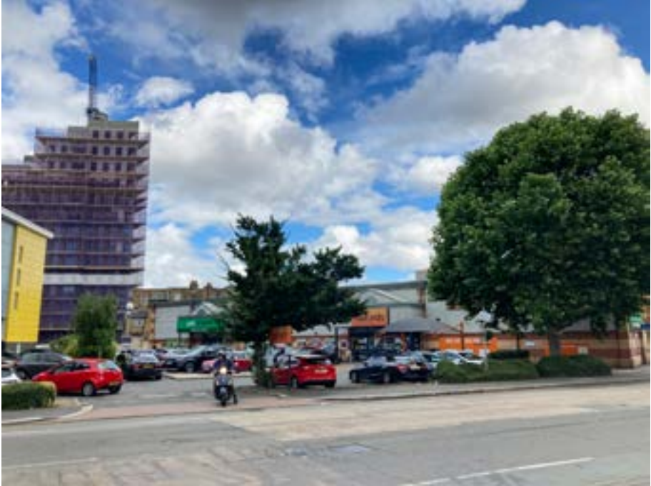
4. View of existing car park to Lombard Road
