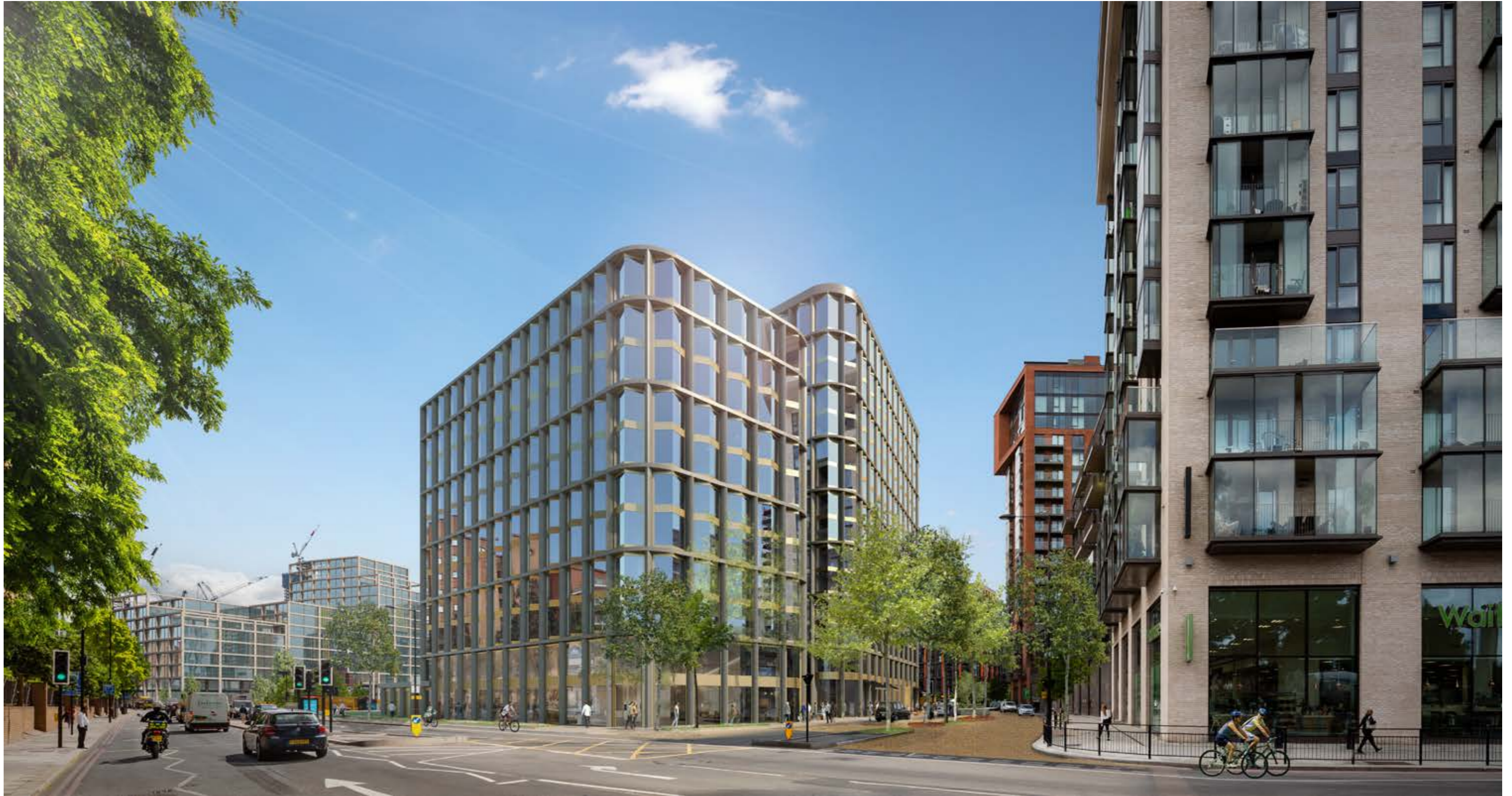
Proposed View from Nine Elms Lane / Ponton Road
